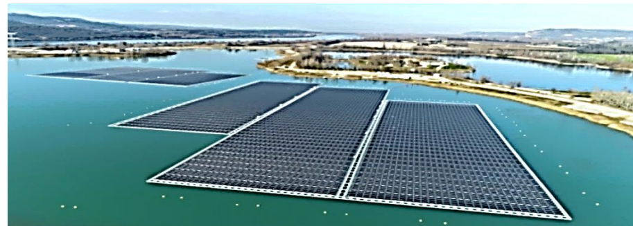
The largest floating solar farm in Europe
